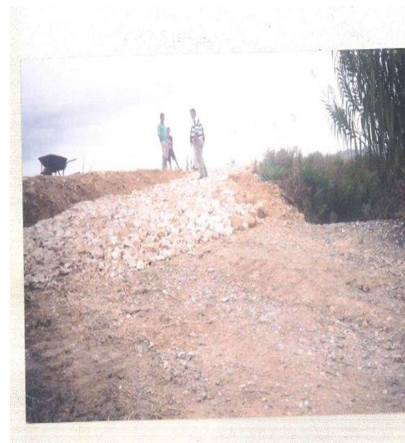
Photo: Placing stone belts
