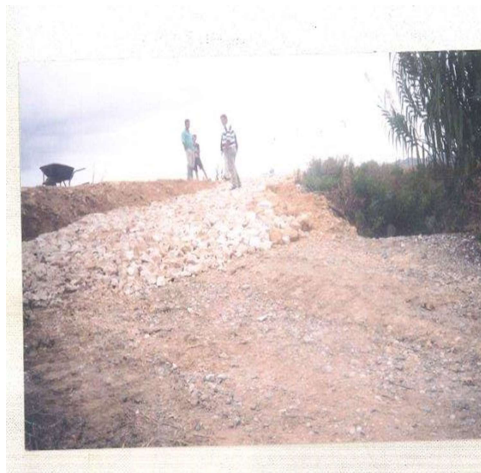
Photo no : embankments protection
